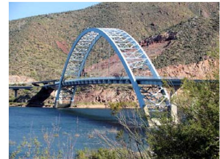
Scenic bridge over Roosevelt Lake near Globe
